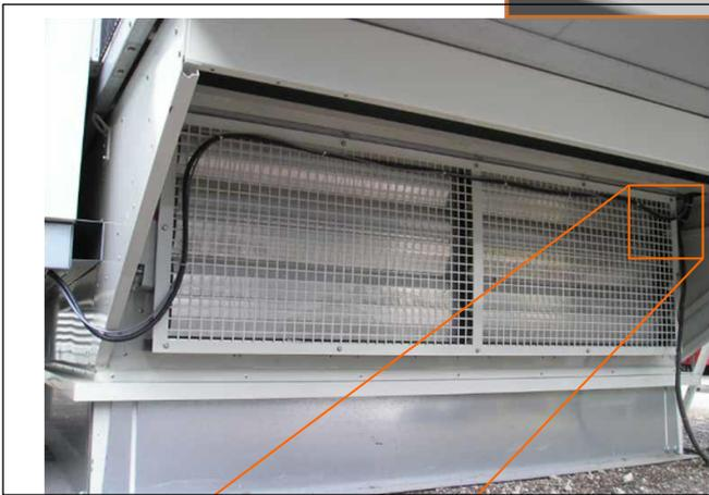
Then, attach the 2 cables to the grid of the extraction curb and insert them into the rooftop electrical panel.
