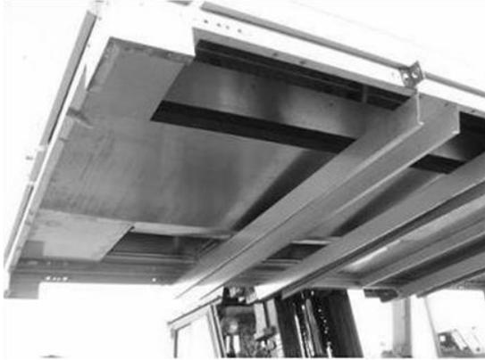
**REMOVE THE FORKLIFT PROTECTIONS BEFORE INSTALLATION**
